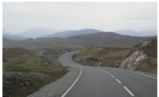
New road construction using ROADEX technologies in the Western Isles, Scotland. (photo: Ron Munro)
