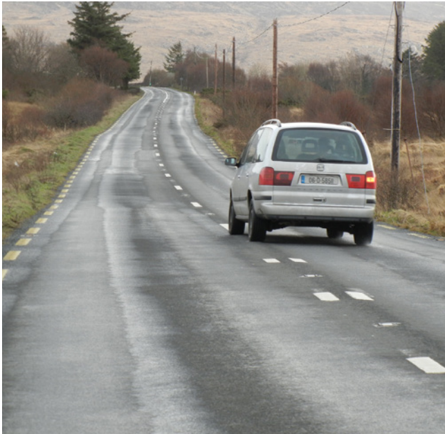
Typical 2 lane road over peat in west Ireland. (photo: Haraldur Sigursteinsson)
