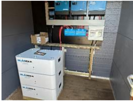
Figure 6 Solar energy system for a summer house complex in Illugastaðir.
