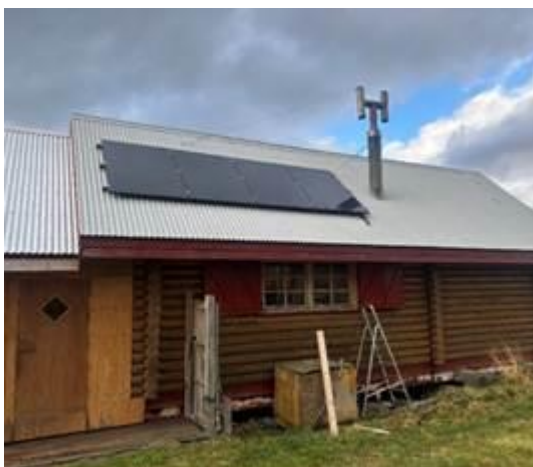
Figure 10 Solar energy system at the summer house Siglunes 3 at Sigulufjörður.
